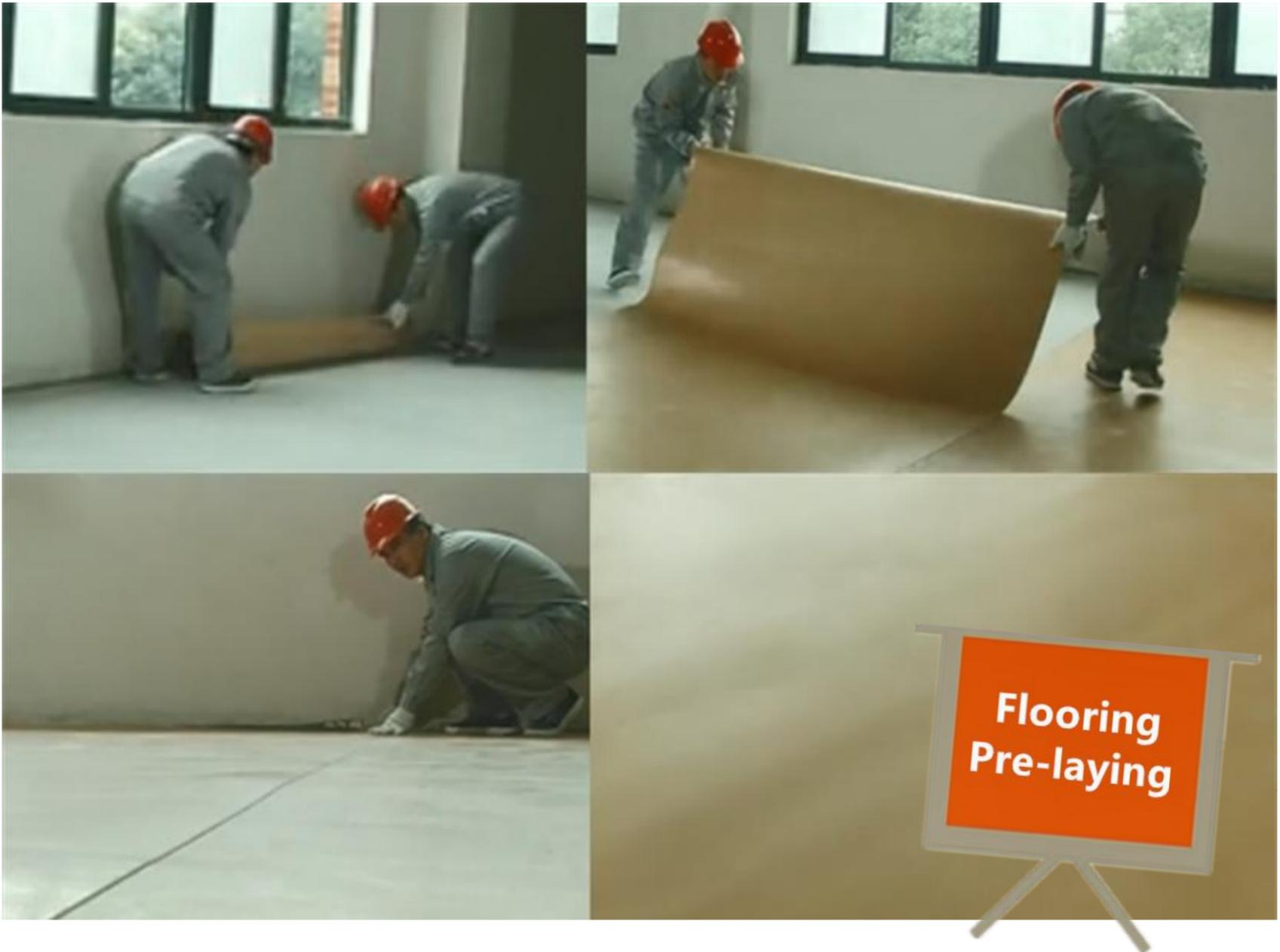
The overlaps of two floors should be cut across, generally requires overlapping 3cm. Using special trimmer to cut and clean the rough edges of the flooring sheet.
