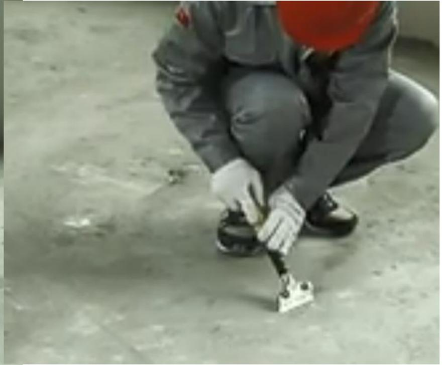
The sanding machine to polish the subfloor with the appropriate grinding disc that is to deal with uneven surface and floating ash.
