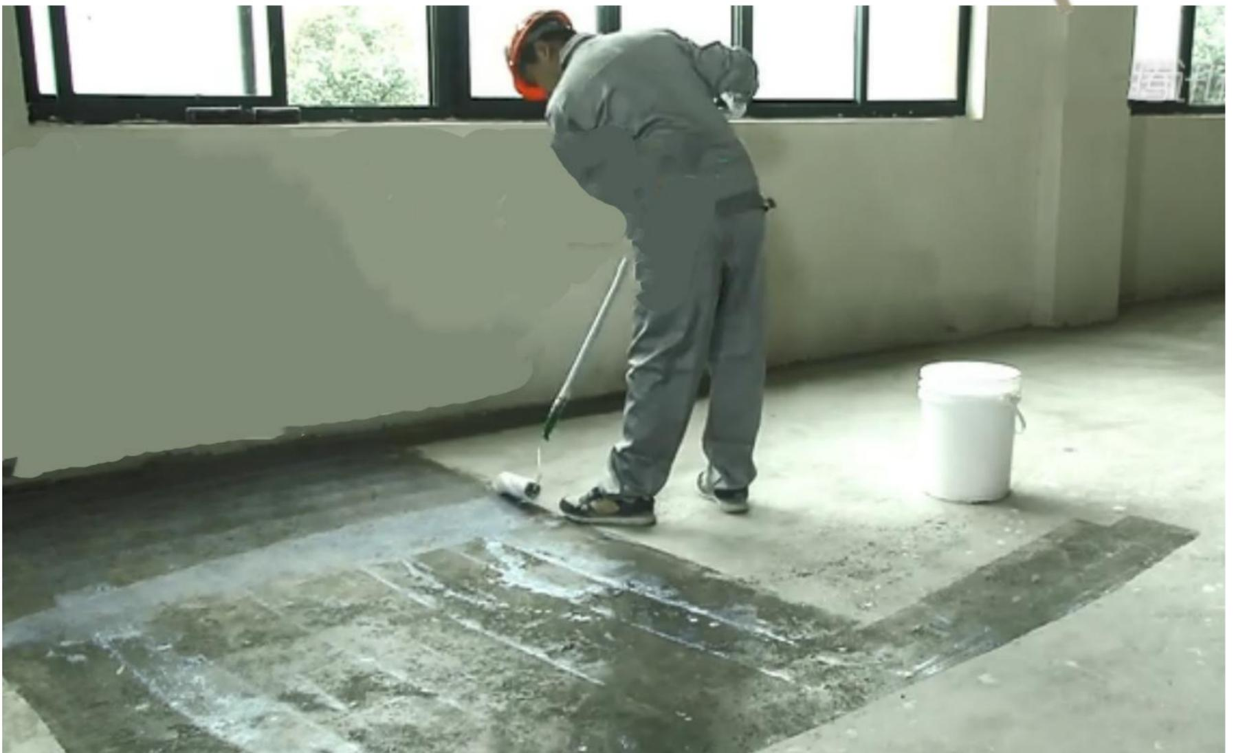
Constructing the interface primer should be uniform without obvious liquid accumulation. After it is dried, self-leveling construction can be carried out.
