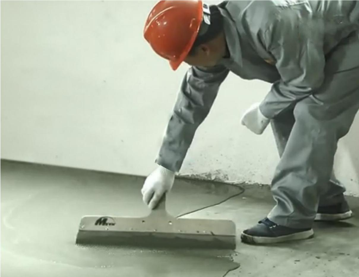
Pouring the stirred cement slurry on the floor, and using the specialized tooth rake scraper and suitable rack to scrap the self-leveling.
